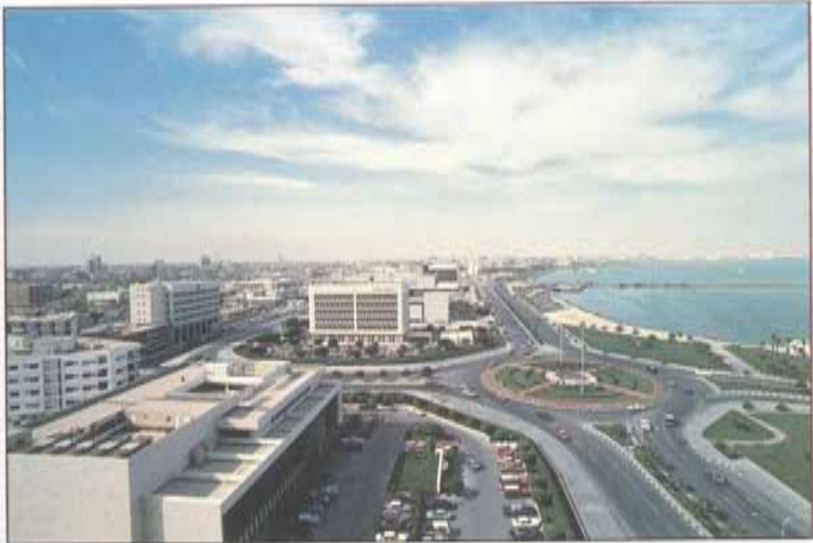
Aerial view of the city of Doha with Qatar National Bank Head Office building along the Corniche.
